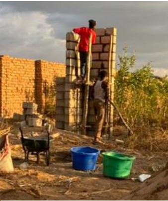
Brick tower to store tank.
